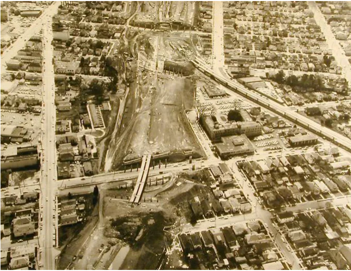
Oakland's Grove Shafter Freeway, 1968, by Russ Reid (Courtesy of Oakland Museum of California)
